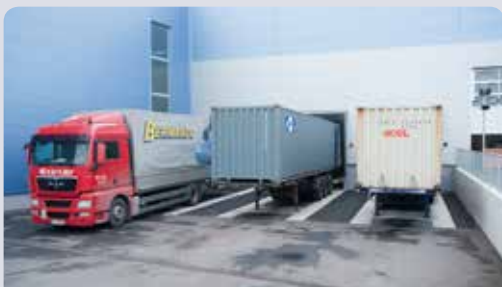
Daily incoming and outgoing goods
